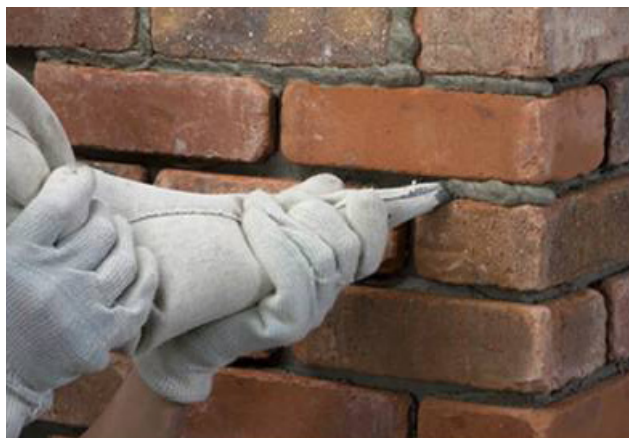
Photo 2 Mortar Placement Using a Grout Bag
