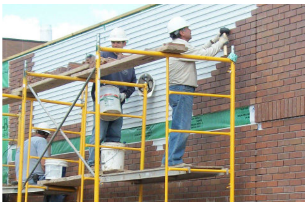
Photo 3 Installation of Modular Panel
