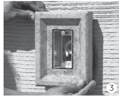
Center electrical box stone over the extension box; level and plumb. Use removable shims if required.
