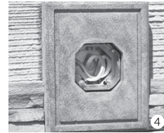
Complete placement of manufactured stone veneer or other exterior material around electrical box stone.
