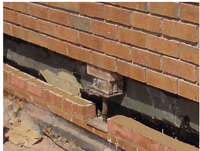
Photo 4 Flashing Installation Using Temporary Support
