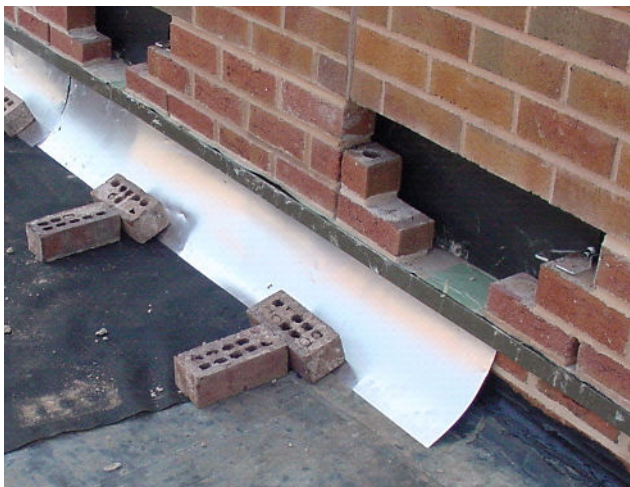
Photo 3 Flashing Installed in Alternating Sections
