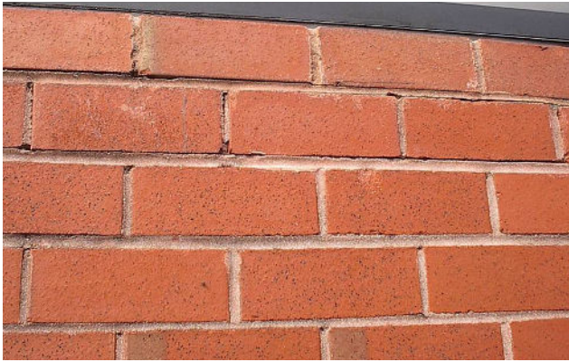
Photo 1 Mortar Joints in Need of Repointing
