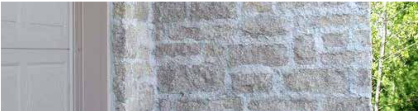
Concave mortar joint
