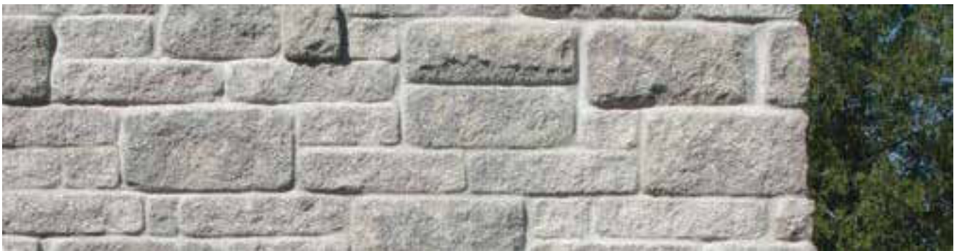
Concave mortar joint
