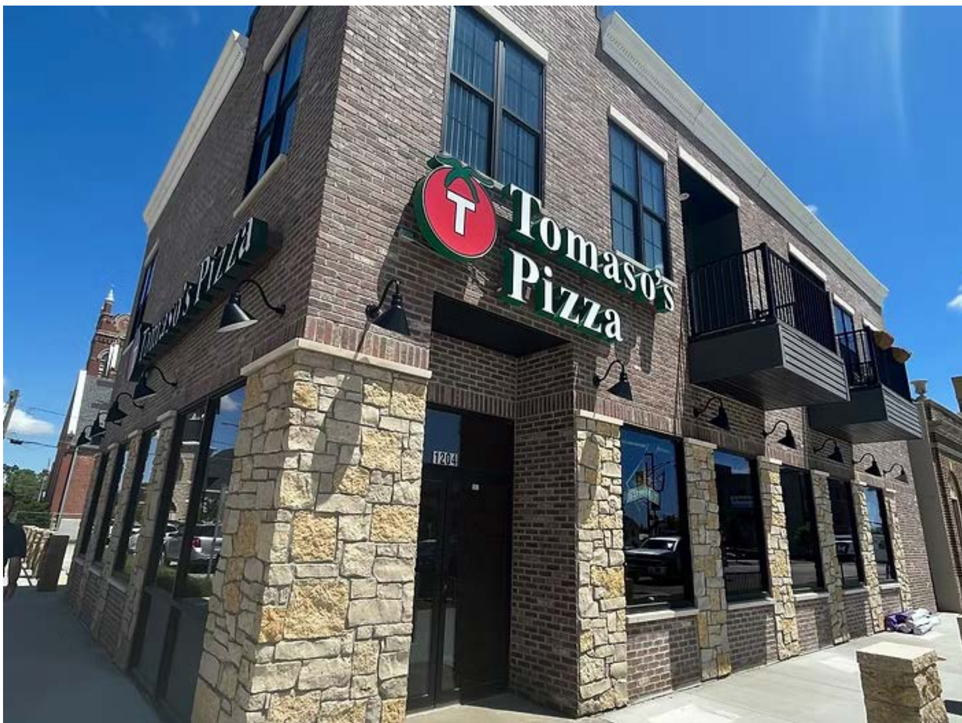
Tomaso's Pizza - Cedar Rapids, Iowa Installation Product - Speedymason Brick Lath Size of Project - Approx 4000 Square Feet
