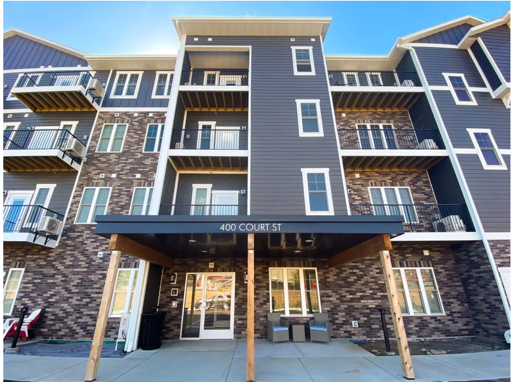
Great River Residence - Onalaska, Wisconsin Installation Product - Speedymason Brick Lath Size of Project - 9,330 Square Feet
