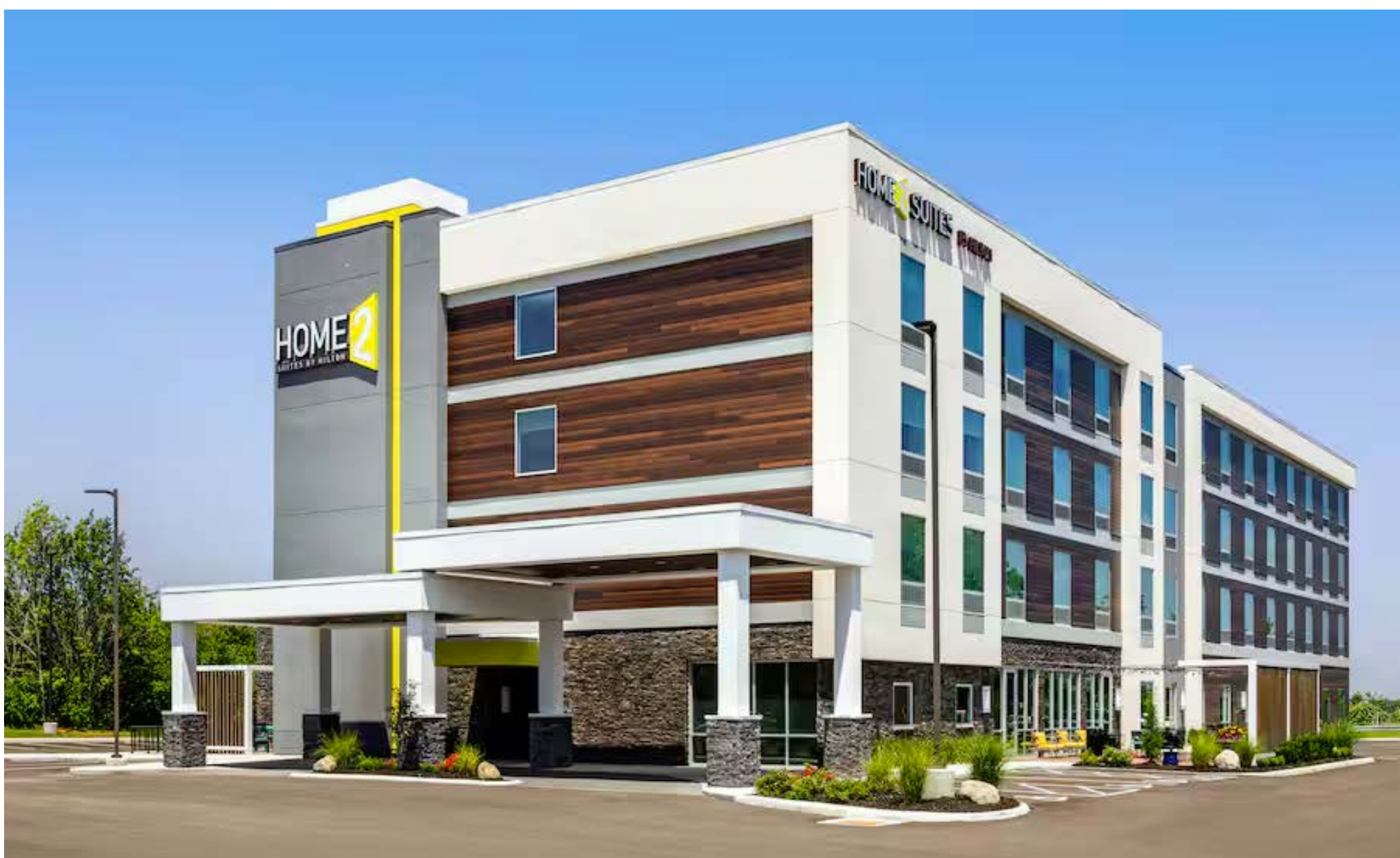
Home 2 - Columbus Ohio Installation Product - Stone Lath Size of Project - 2800 Square Feet
