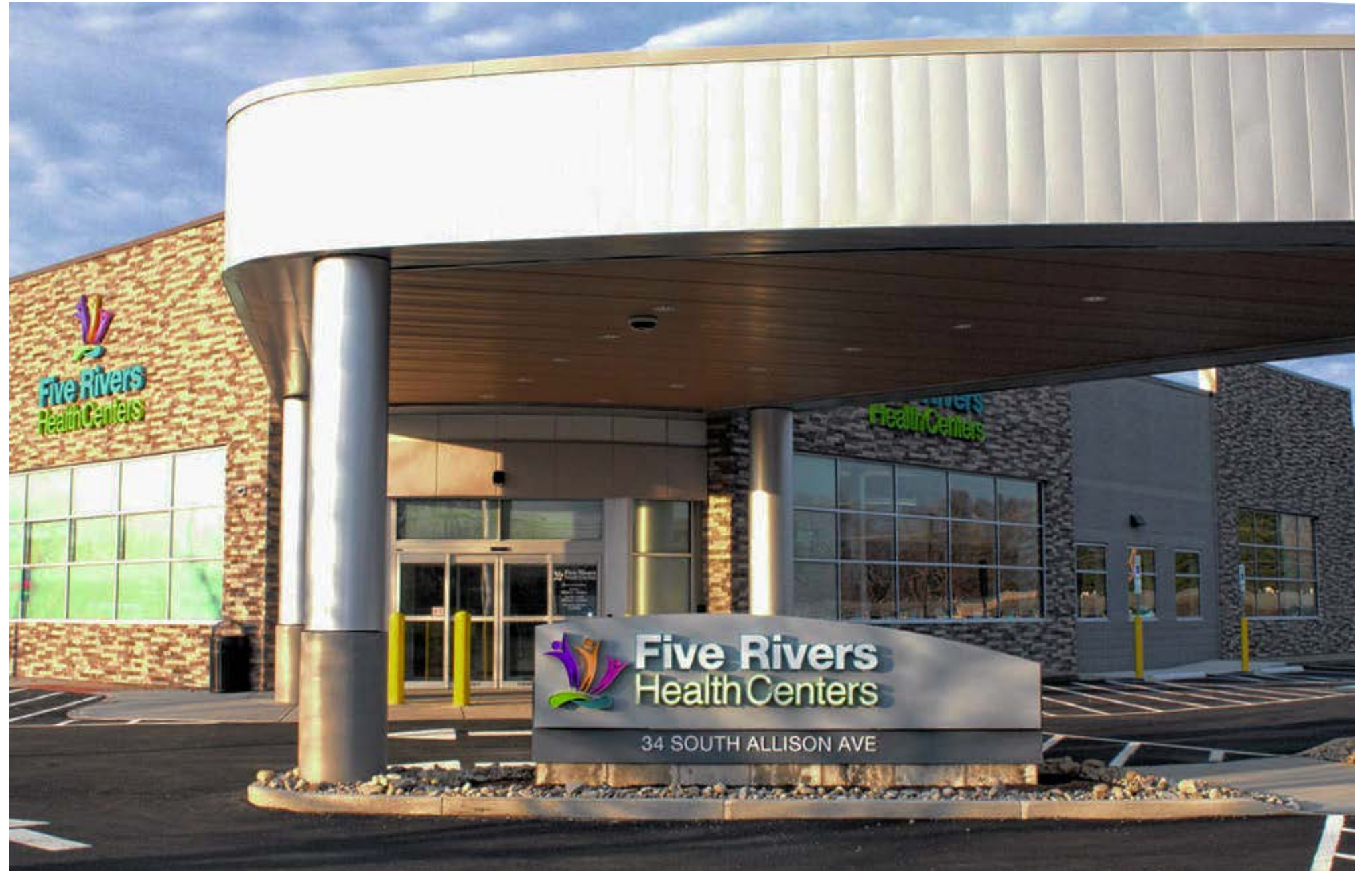
Five Rivers Health Centers - Xenia Ohio Installation Product - Brick Lath Size of Project - 3000 Square Feet
