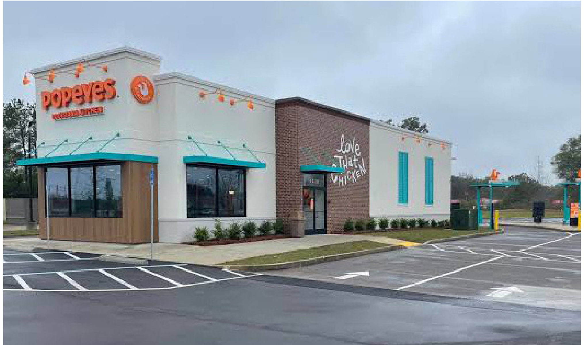
Popeyes - Cincinnati Ohio Installation Product - Brick Lath Size of Project - Approx 3000 Square Feet
