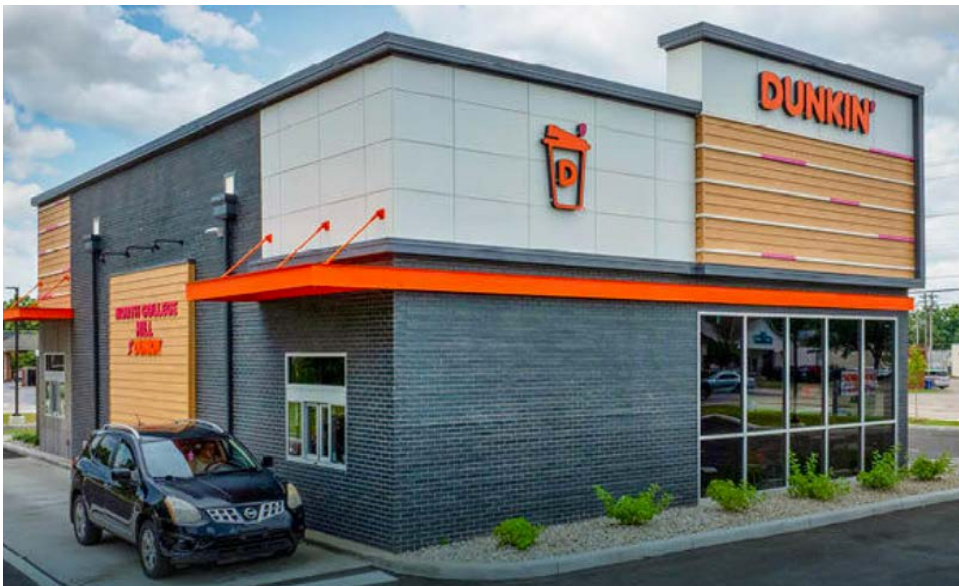
Dunkin' Donuts - Cincinnati Ohio Installation Product - Brick Lath Size of Project - 2500 Square Feet
