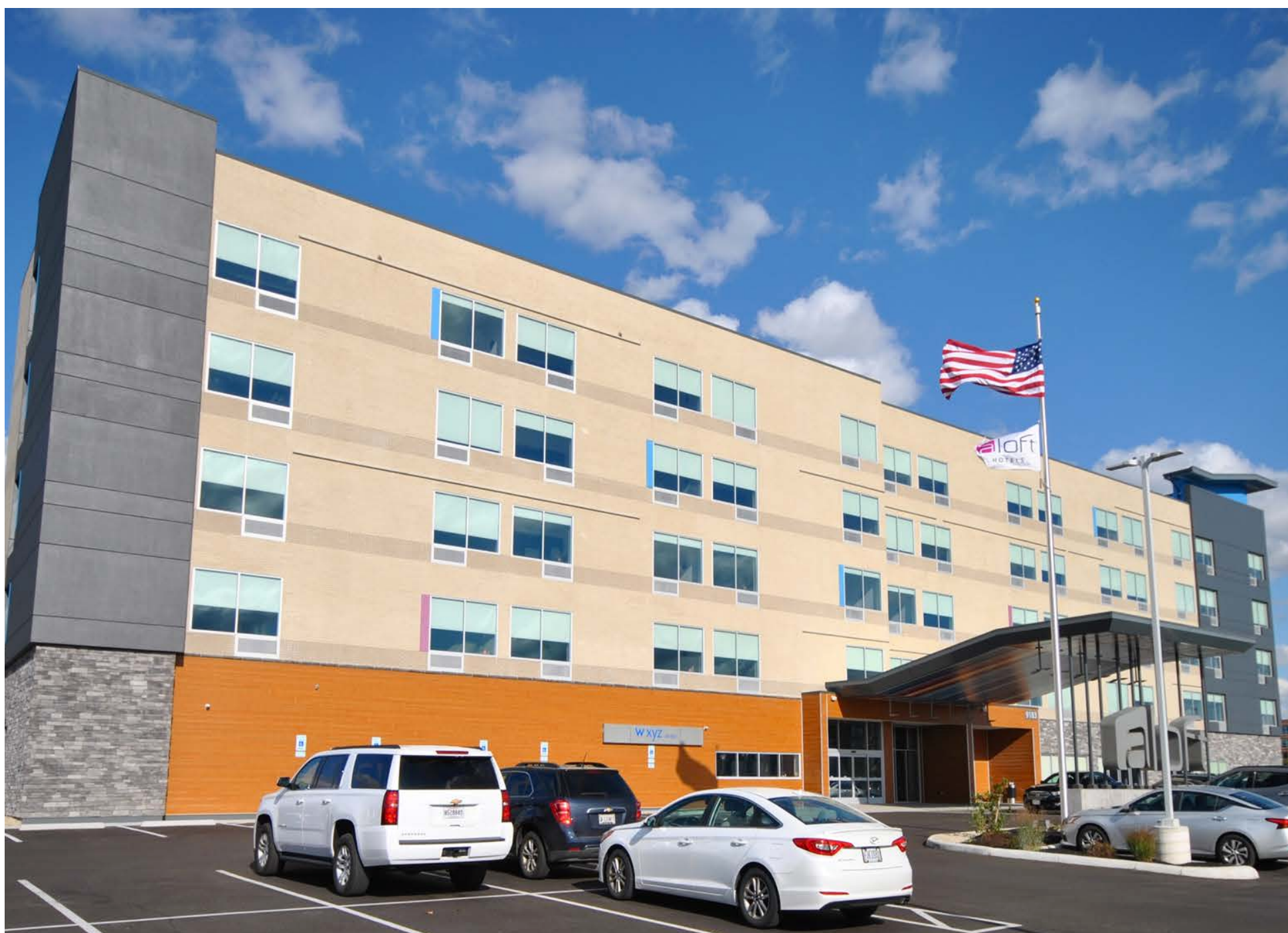
Aloft Hotel - West Chester, Ohio Installation Product - Speedymason Brick Lath and Stone Lath Size of project - 19,894 Square Feet of Thin Brick and 7,400 Square feet of Stone Veneer
